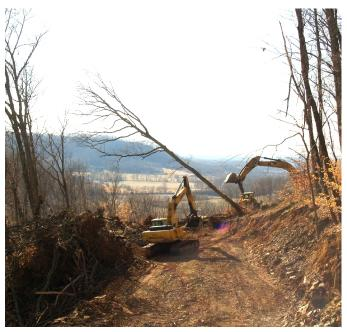
The Walker Company is primarily using heavy equipment to clear the haul road, borrow areas, and storm water management features.
